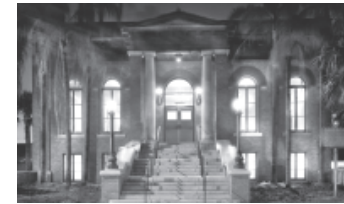
The newly refurbished West Tampa Library
