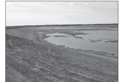
Recent photo of Tampa Bay Water's nearly-empty 15-billion gallon reservoir
