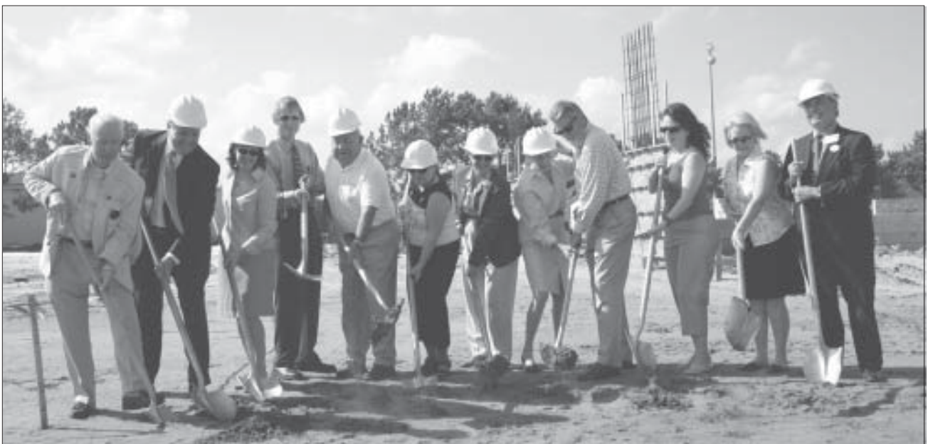
County Commissioners joined with representatives from the SouthShore Roundtable, county staff and the project contractor and architect to break ground on the new South County Regional Service Center in Ruskin. This center, which is scheduled to open in fall 2005, will house offices of the Citizen Action Center, the Clerk of the Circuit Court, Code Enforcement, Planning and Growth Management, the Property Appraiser's Office, the South Shore Justice Center and the Water Department.
