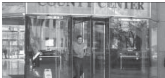
Sliding doors will soon replace this revolving glass entry, allowing for easier access.
