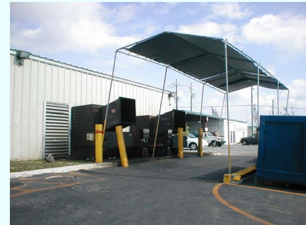
Ft Lauderdale Airport's on-site recycling facility
