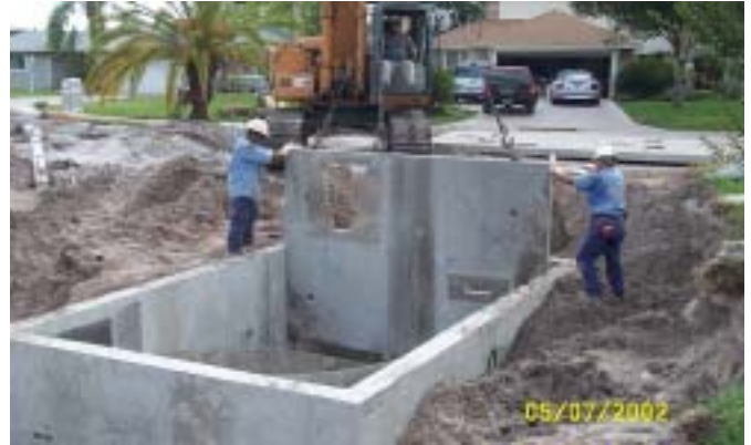
Inserting a Baffle Wall
