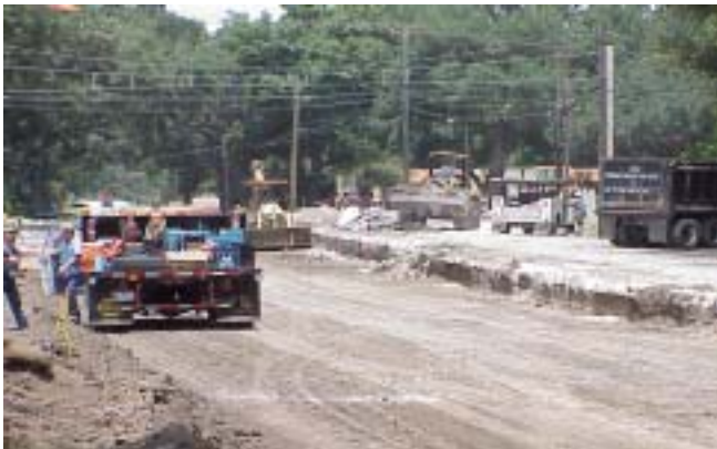
Lithia-Pinecrest and Bryan Road Intersection
