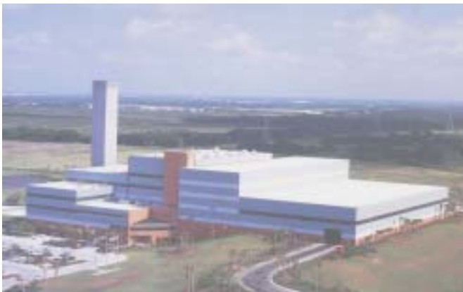
Resource Recovery Facility
