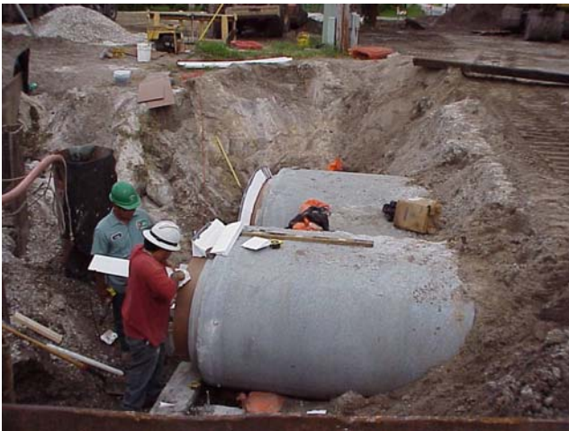
Workers installing Reinforced Concrete Pipe
