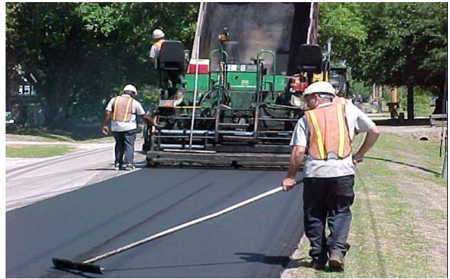
County Workers Resurfacing Road
