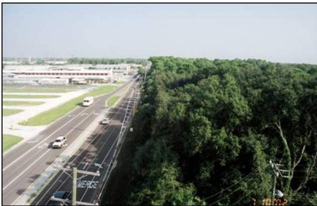
Racetrack Road (Before Improvements)
