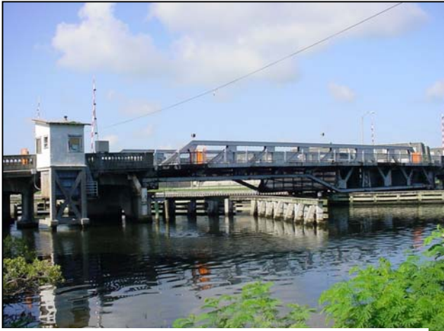
The Columbus Ave. Bridge over the Hillsborough River
