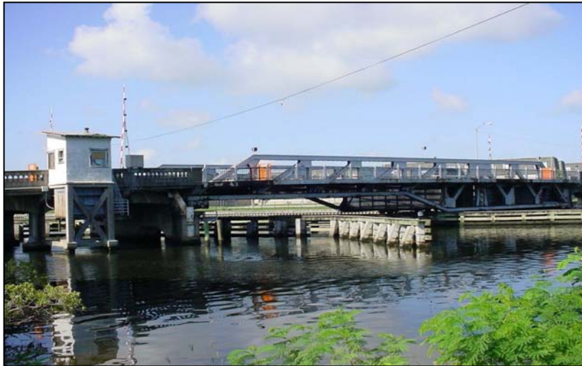
Columbus Drive Bridge over the Hillsborough River
