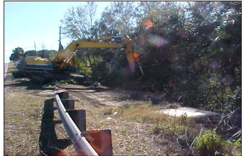
Symmes Road Bridge Improvements
