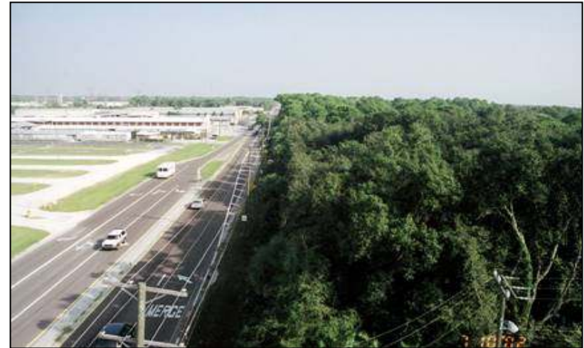
Racetrack Road (Before Improvements)
