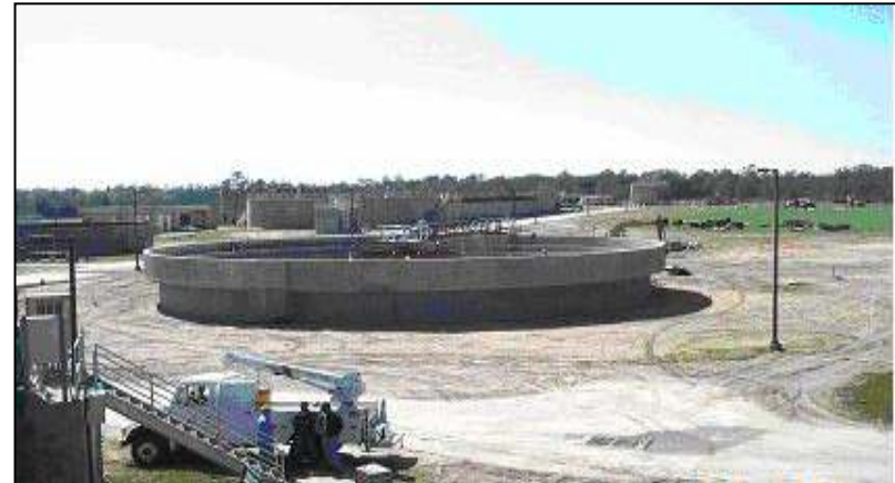
Valrico Advanced Water Treatment Plant Expansion
