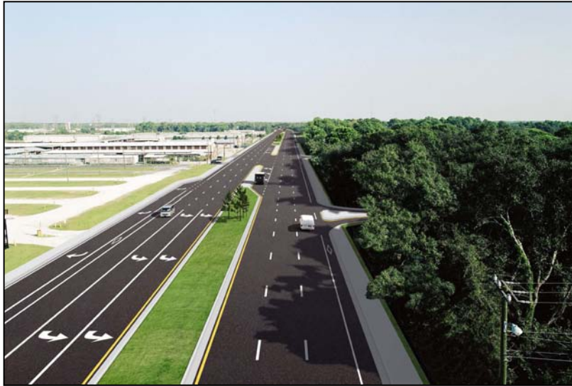
Racetrack Road (After Improvements)
