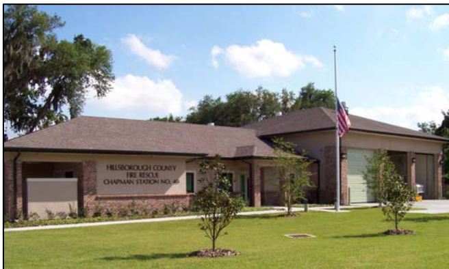
The Chapman Fire Station is a prototype of future three-bay fire stations included in this Program.
