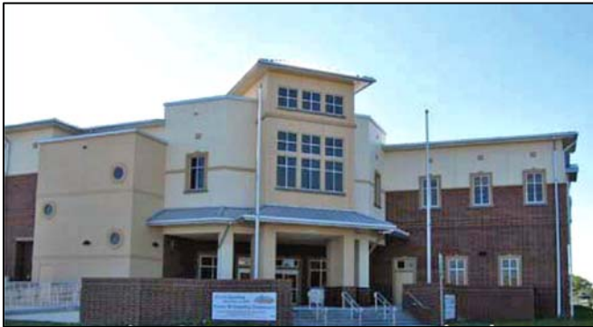
Completed in FY 09, the Town and Country Commons Regional Library is co-located with a senior citizen center and a Headstart Center and includes a playground and park features.
