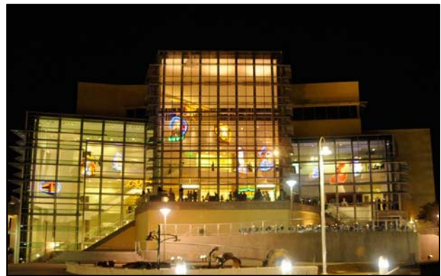
The Tampa Bay History Center is the County's first new LEED-certified "green" building and features the unique history of the region.
