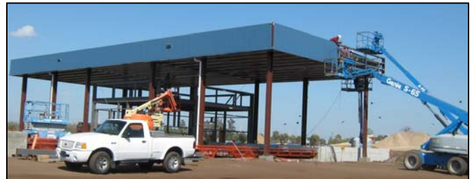
Construction of this entrance canopy is just one of many improvements being made to the South County Transfer Station.
