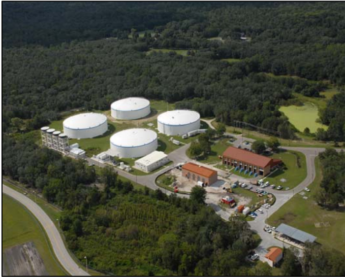
Lithia Water Treatment Plant - Lithia Auxiliary Power Improvements Project
