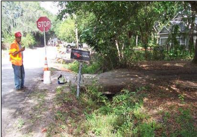
Otto Road Drainage Improvements will be completed in FY 10.
