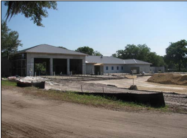
University Area Fire Station #14 (Under Construction)
