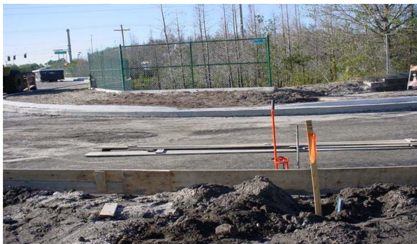
Zambito Road Realignment
