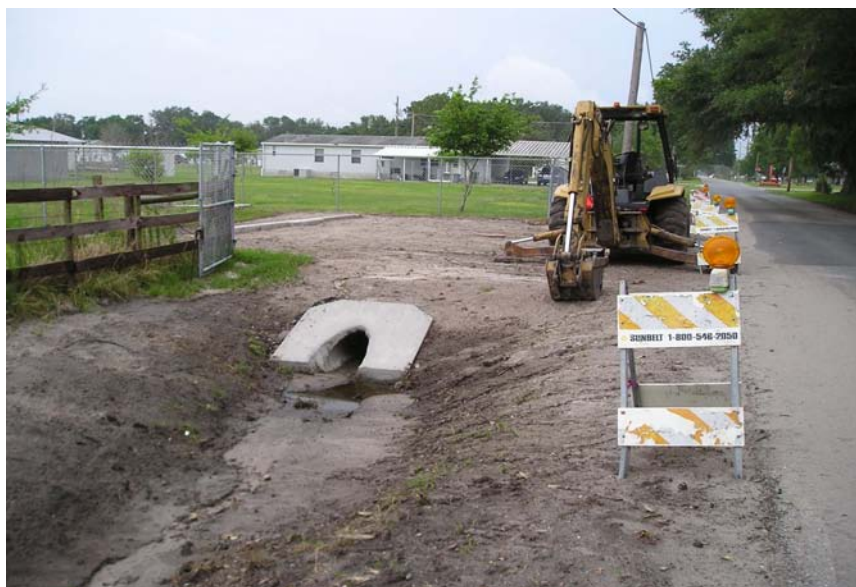
Clay Turner Road Stormwater Improvements
