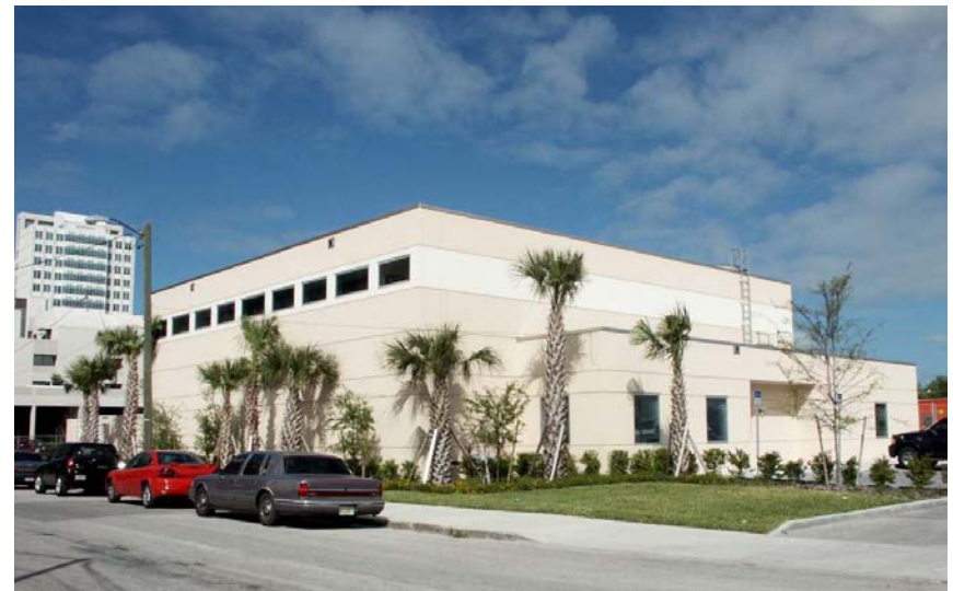
New Chiller Plant
