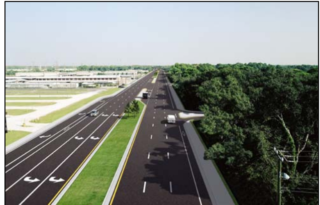
Racetrack Road (After Improvements)
