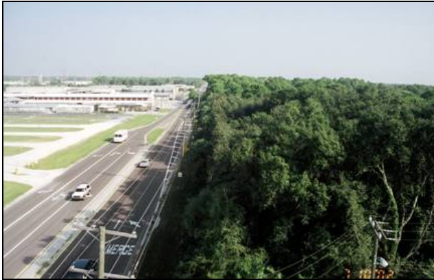
Racetrack Road (Before Improvements)
