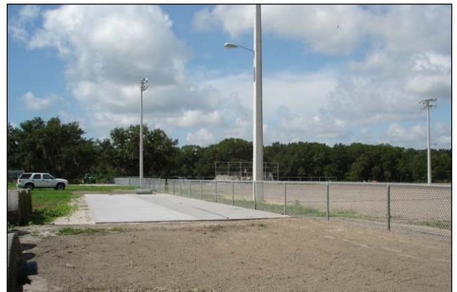
The estimated cost of William Owen Pass Park Improvements project is $3.5 million
