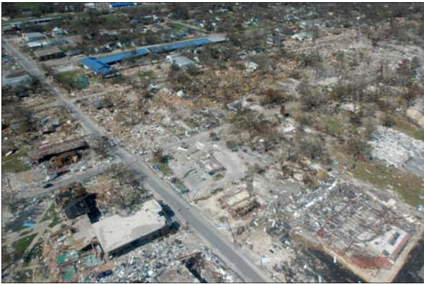
Hurricane Katrina Damage in Gulfport, Mississippi
