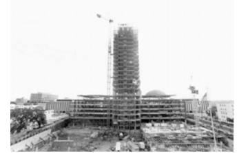
Florida's Current Capitol Under Construction in the 1970's
