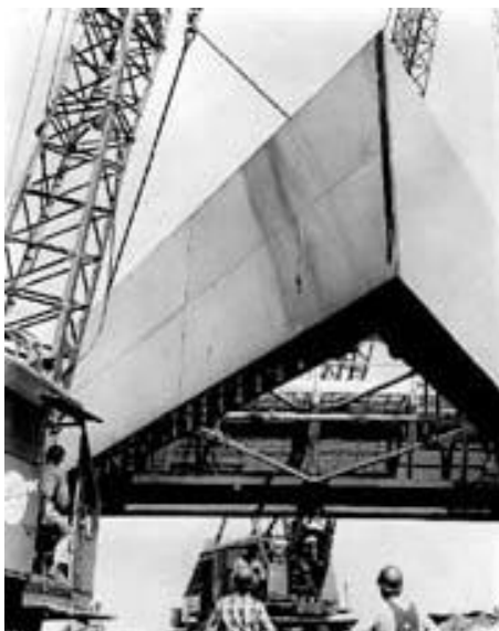
Fig. 1, Crawler cranes place the first 72 Feet
