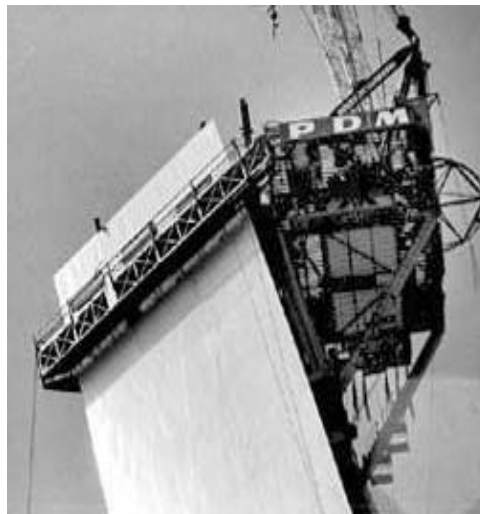
Fig. 2, Climbing cranes on the back of the cantilevers.
