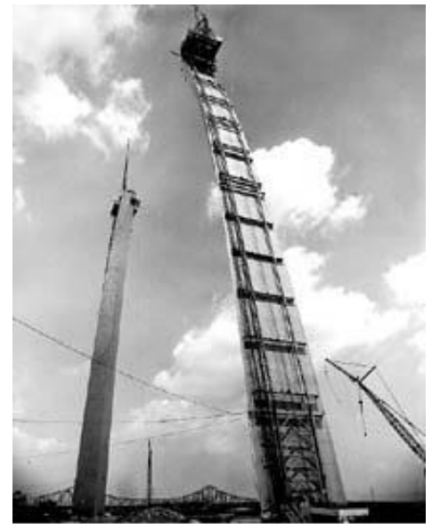
Fig. 3, The workmen' elevator car would rise up the creeper derrick track.
