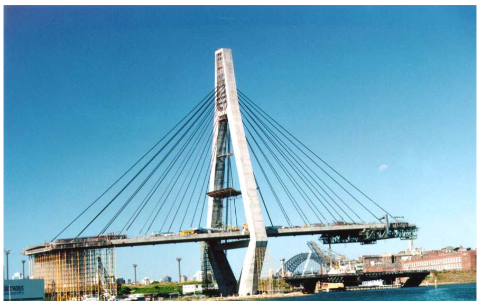
FIGURE 3: WESTERN TOWER CONSTRUCTION SEEN FROM GLEBE ISLAND.
