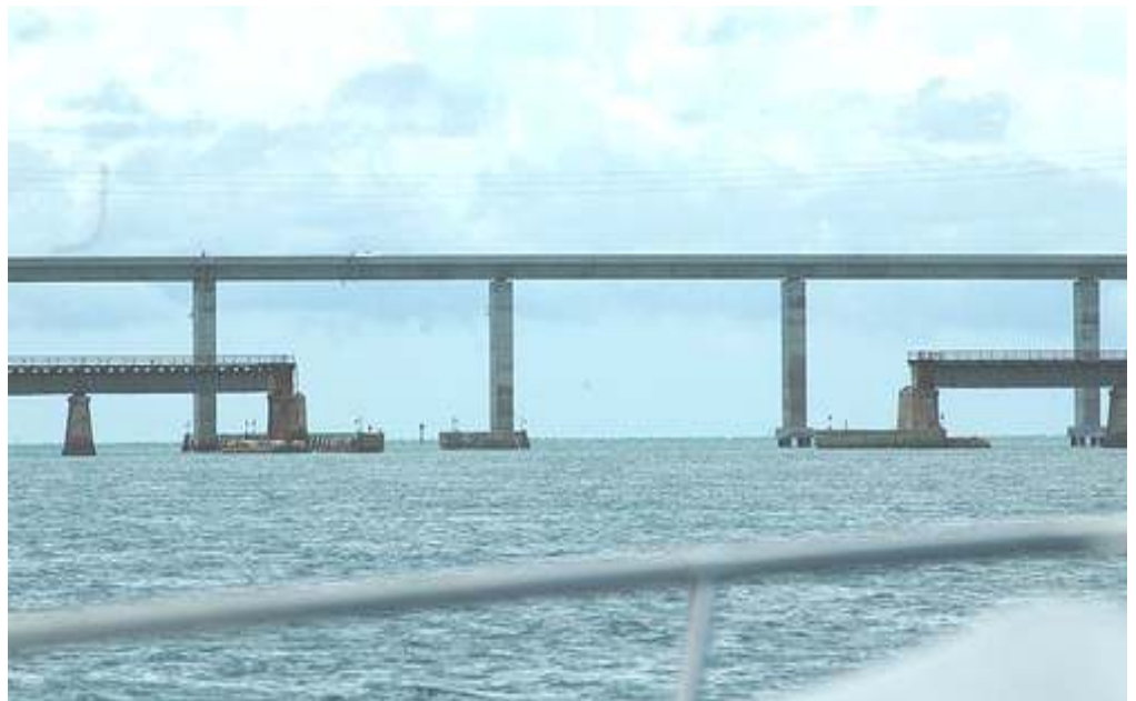
FIGURE 3: 65' vertical clearance of new bridge at Moser Channel with old bridge, foreground, having swing span permanently removed
