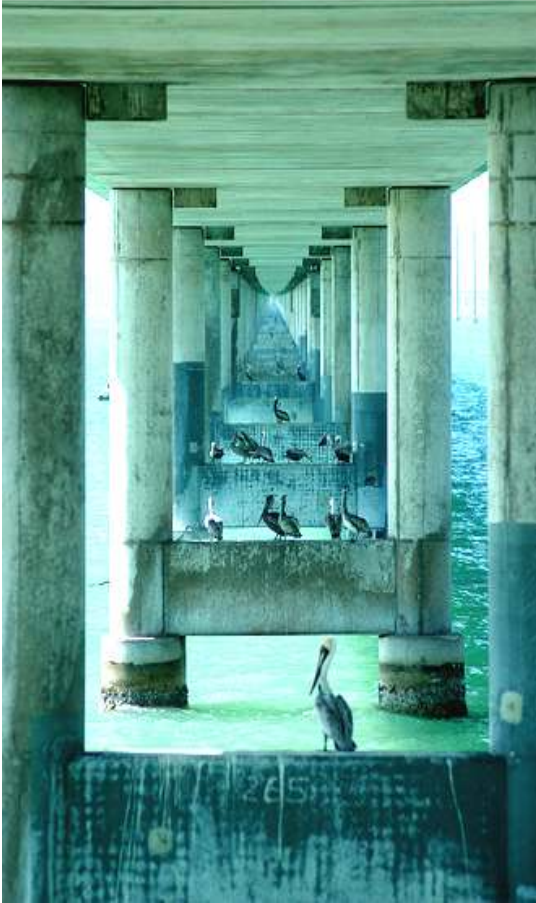
FIGURE 4: 5.5 miles of level spans on 3' diameter concrete shafts.
