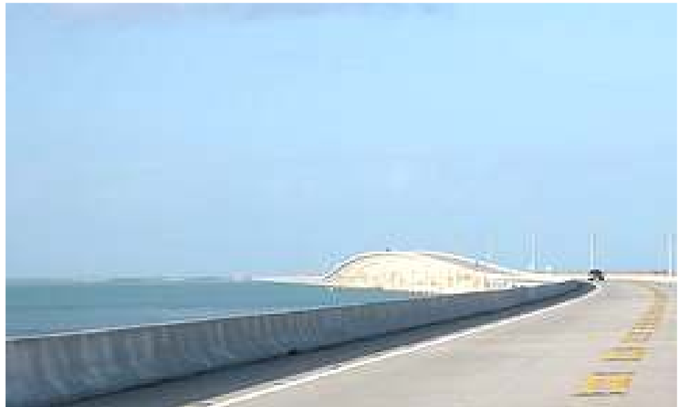
FIGURE 5: One mile vertical curve on box piers over Intercoastal Waterway.
