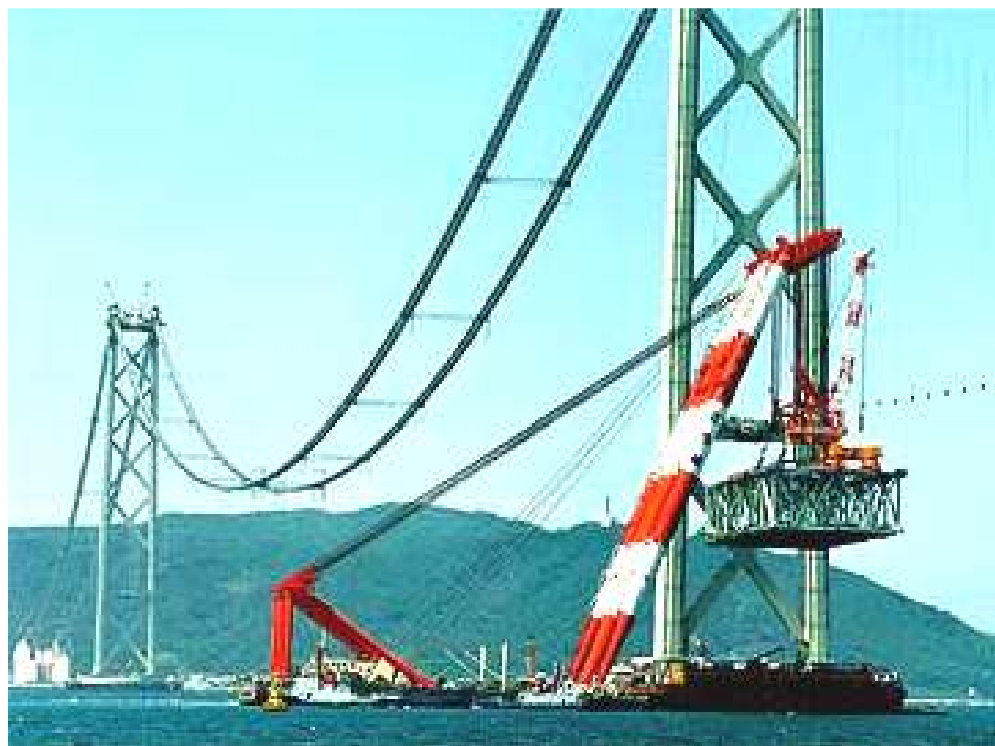
FIGURE 3: Limber configuration at time of '95 Kobe quake minimized impact
