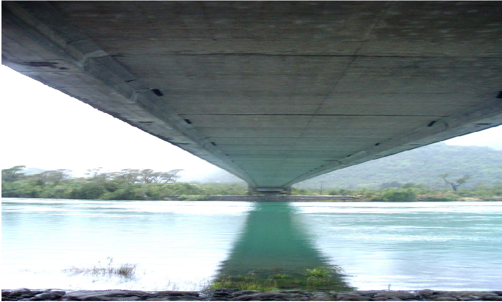
FIGURE 5: Yelcho Bridge carries road over river to edge of Andean glacier
