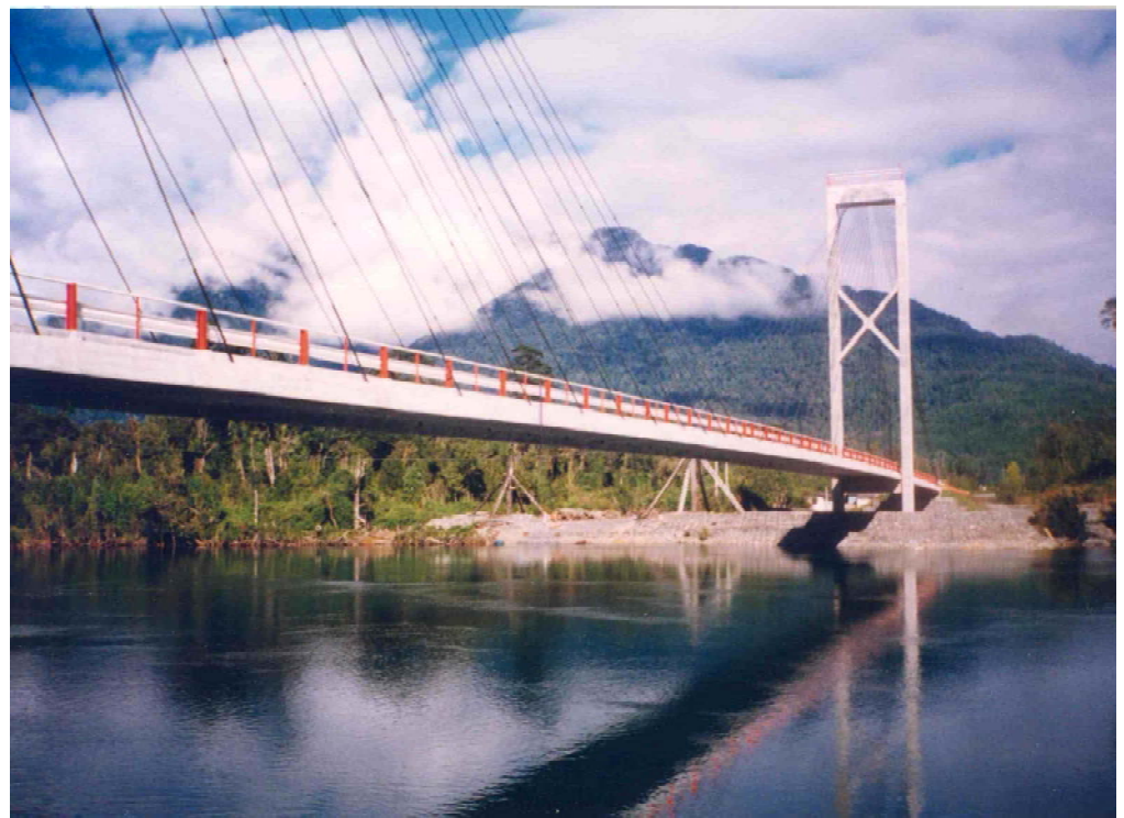
FIGURE 6: The first cable-stayed bridge in Chile spans the Yelcho River
