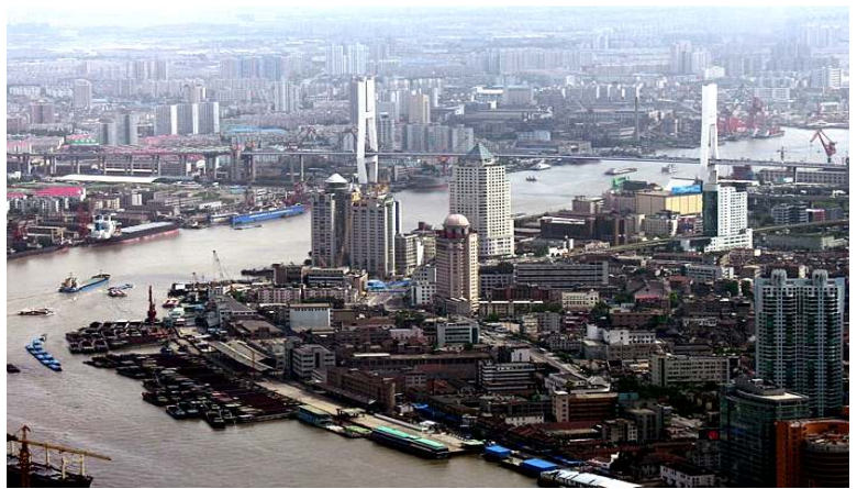
FIGURE 2: View south with Nanpu Bridge reaching to east shore beyond
