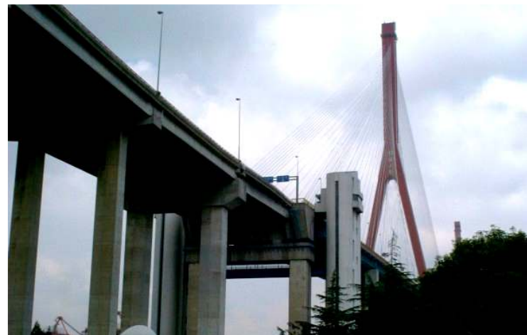
FIGURE 7: Ground view of Yangpu elevator towers
