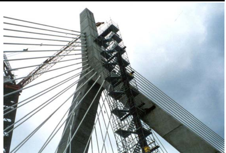
Attaching tension members of the Zakim Bunker Hill Bridge in Boston
