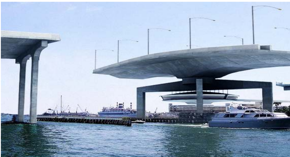
FIGURE 7: North elevation of concept's open, swings-pan, pivot-point with suspended restaurant
