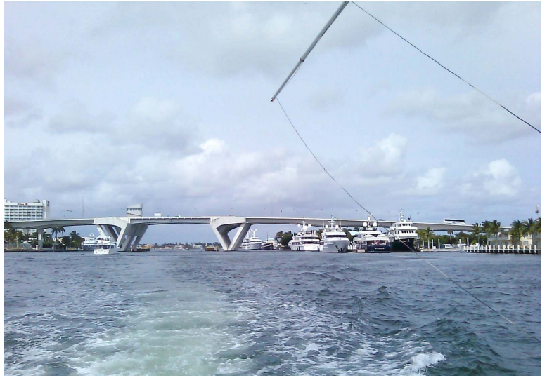
FIGURE 6: Water level, south elevation, of existing bridge
