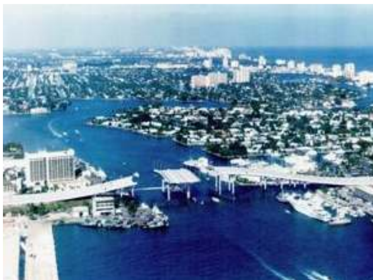
FIGURE 2 : View of concept with swing span open
