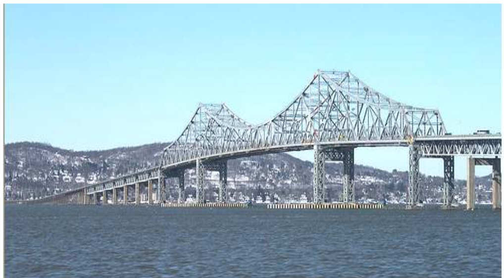
FIGURE 5: The seven lane Tappan Zee Bridge today viewed from the east shore
