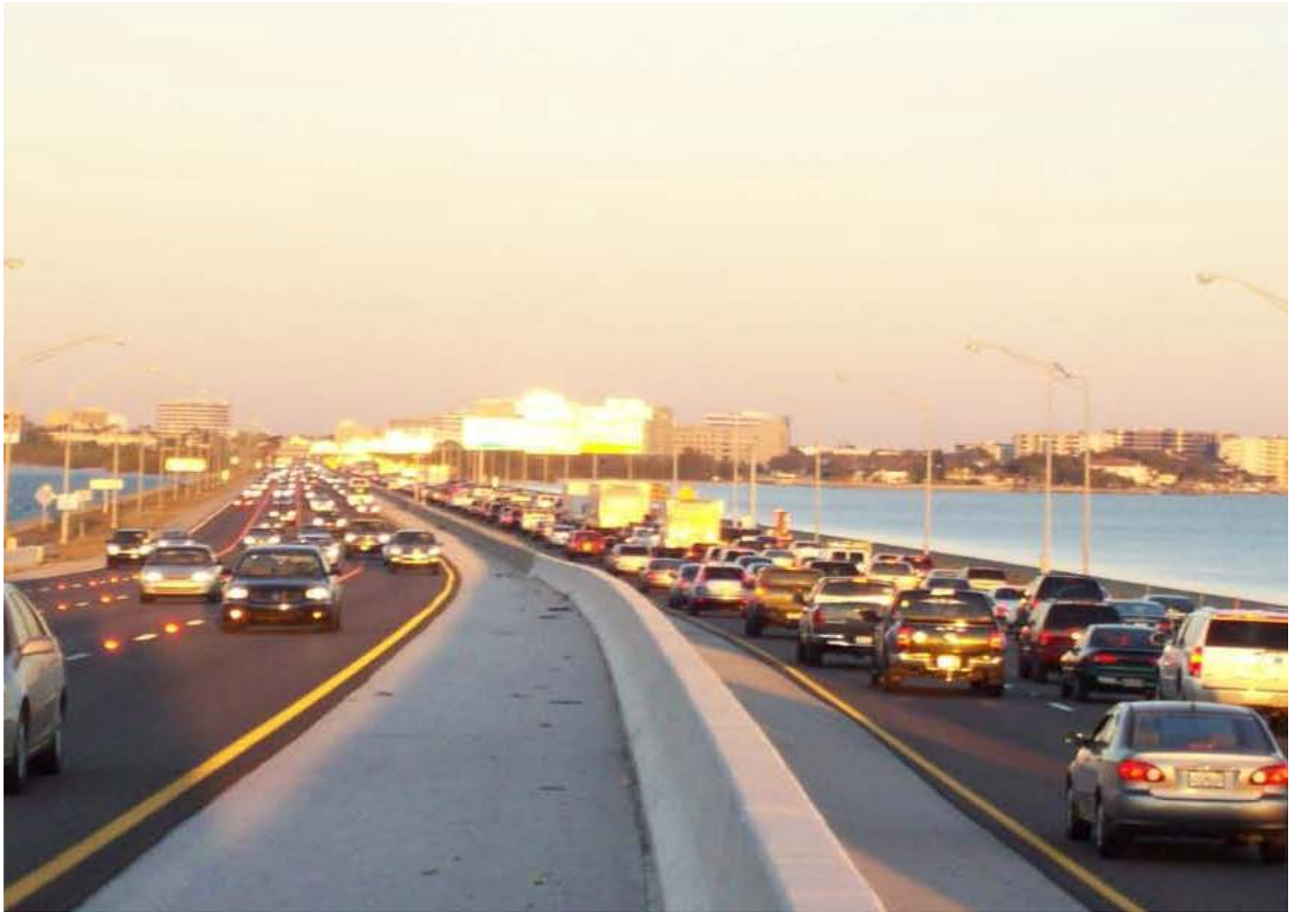
I-275 West, Looking East
