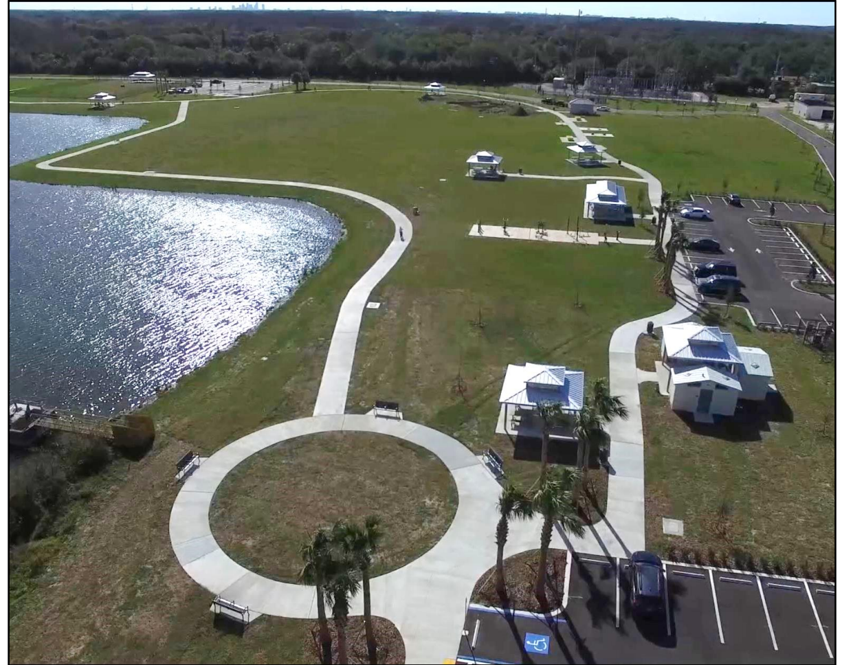
Aerial South View – Photography 1/12/19
